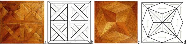
Fig. 1. Tile from the Master's Study (a - tile view, b - pattern and fibre direction) and from the Salon of the State Apartment (c - tile view, d - pattern and fibre direction).
