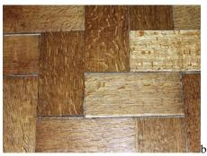
Fig. 10. Example of a plank from the Rococo Salon showing the difference in thickness and the gaps that appeared as a result of wood shrinkage and an example of their compensation with wooden battens.
