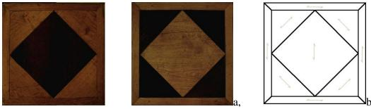
Fig. 4. Tile from the Bathroom of the State Apartment (a - tile view, b - tile design and fibre direction).
