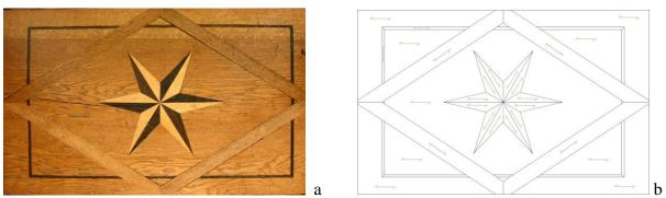
Fig. 5. Tile from the Ball Room (a - tile view, b - design and fibre direction).
