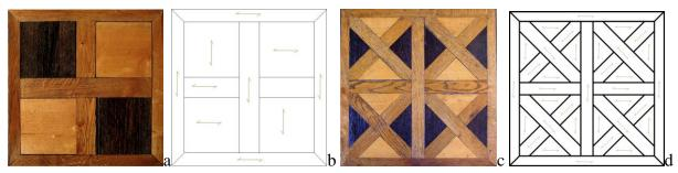
Fig. 2. Tile from the Sculpture Gallery (a - tile view, b - pattern and fibre direction) and the Chapel (c - tile view, d - pattern and fibre direction).
