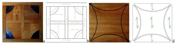
Fig. 3. Tile from the Entrance Salon (a - tile view, b - pattern and fibre direction) and the Bachelor's Apartment (c - tile view, d - pattern and fibre direction).
